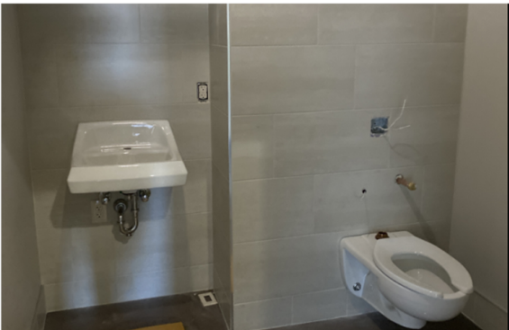
Bathroom Fixtures & Tiling Complete
