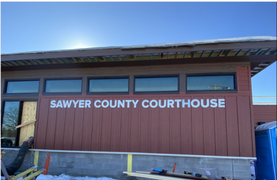
Phase 1 Siding Complete
