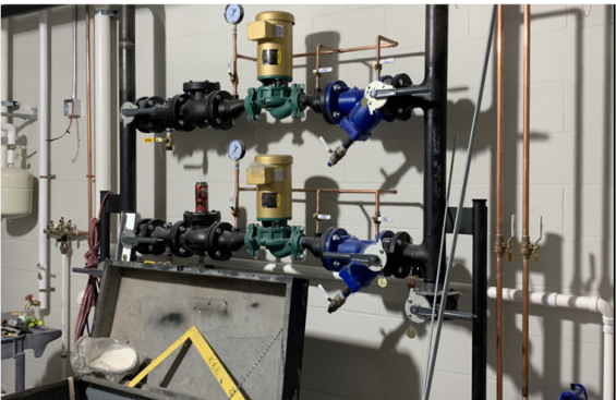
Mechanical Piping Progress
