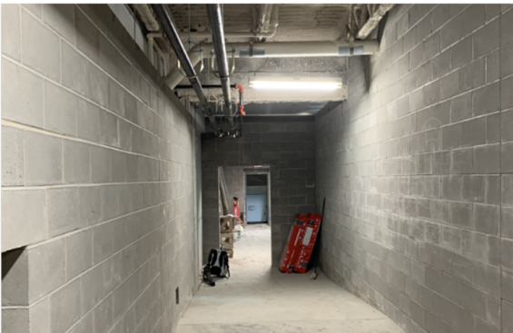
Jail Area CMU Complete
