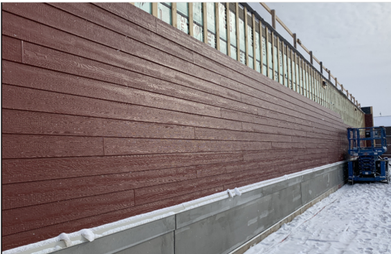
West Elevation Siding Progress
