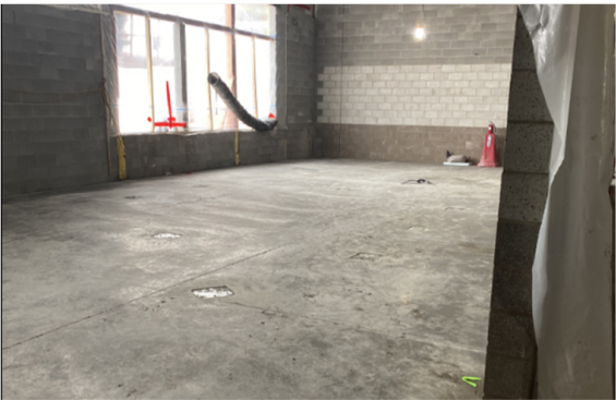
Board Room Slab on Grade Poured
