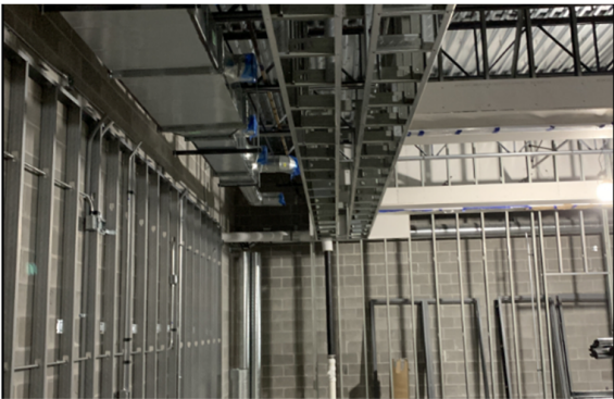
North Courtroom Stud Framing Progress
