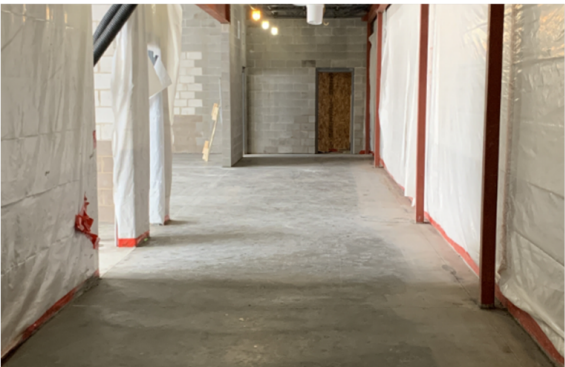
Lobby Slab on Grade Poured
