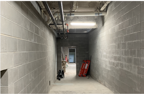
Jail Area CMU Complete
