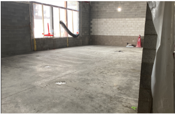
Board Room Slab on Grade Poured
