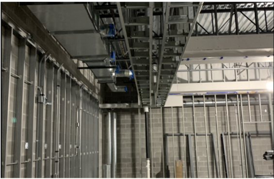
North Courtroom Stud Framing Progress
