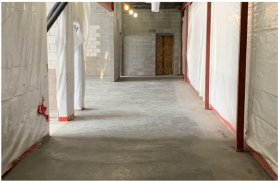
Lobby Slab on Grade Poured
