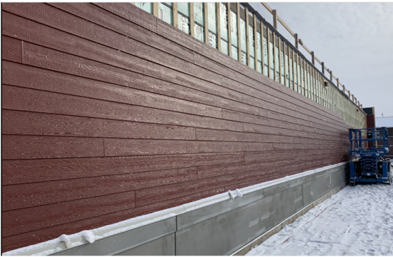
West Elevation Siding Progress
