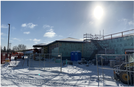
East Elevation Progress
