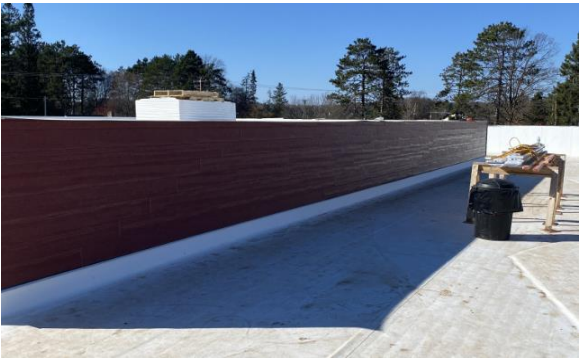
LP Siding Started On High Roof
