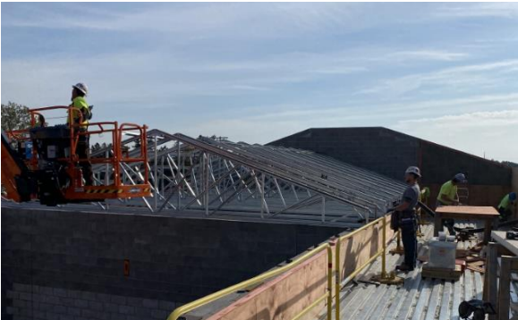
CFM Trusses Progress
