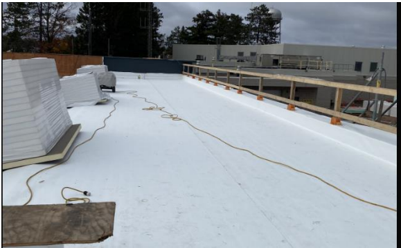
TPO Roofing Completed
