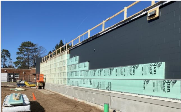
West Elevation Siding Progress
