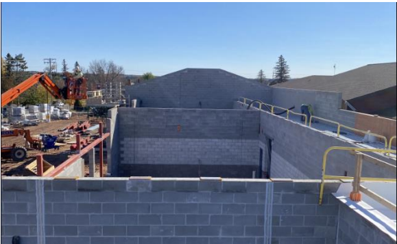
Load Bearing CMU Completed
