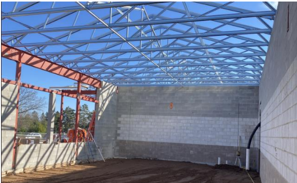
CFM Trusses Set & Structural Steel Complete
