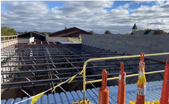
Structural Steel Joist & Deck
