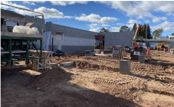
CMU Progress on East Elevation
