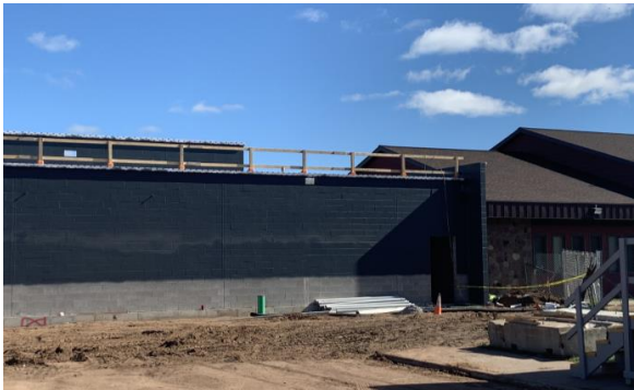
West Elevation Air Barrier
