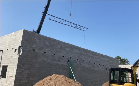
North Courthouse Setting Steel Joist
