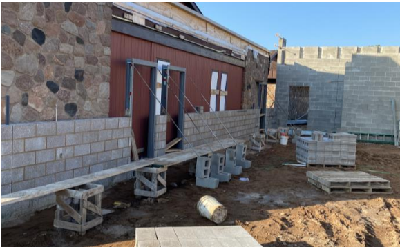
South Firewall Burnished Block Started
