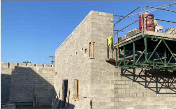
North Courthouse CMU
