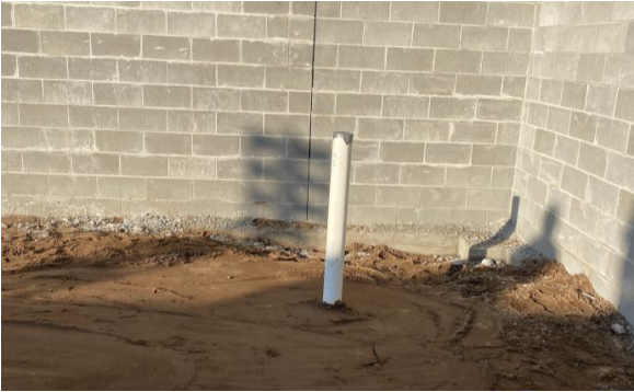
Underground Plumbing Started
