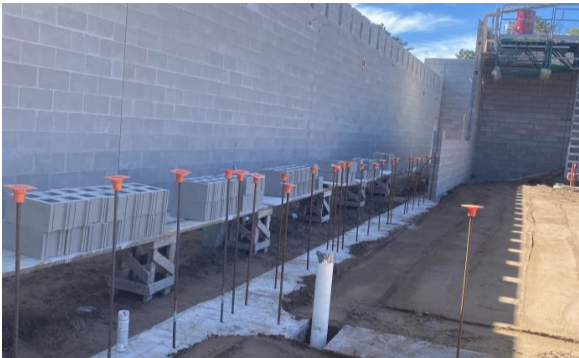
North Courthouse Foundations Complete
