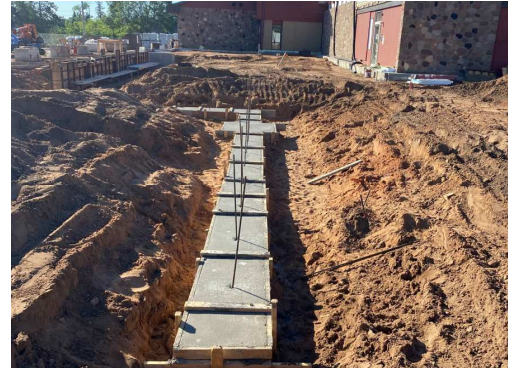
East Exterior Foundation Wall Poured
