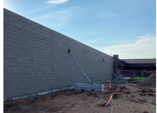
West CMU Wall Complete
