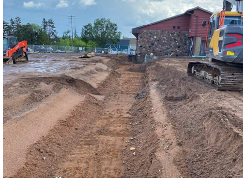
East Exterior Foundation Excavation
