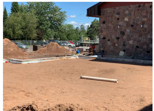
South Foundations Backfilled
