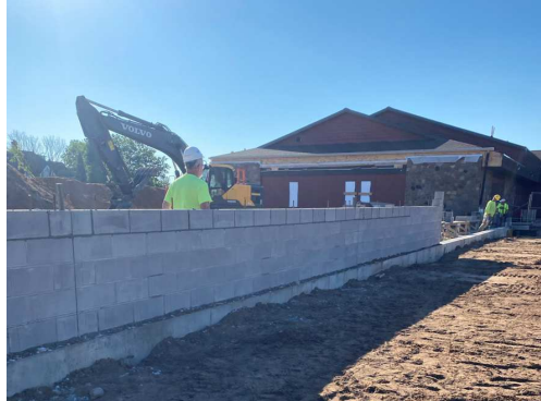
West CMU Wall Started
