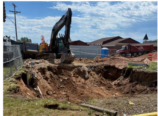
Veteran's Building Demo
