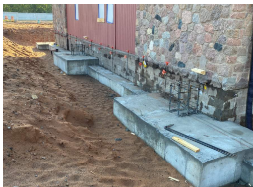
South Firewall Footing Poured
