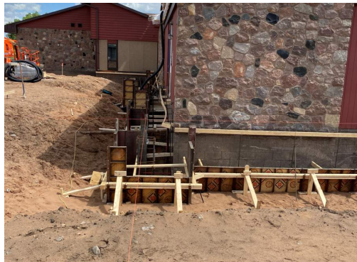
South Firewall Foundations Forming
