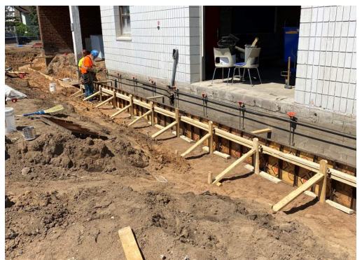
North Firewall Foundations Formed & Poured
