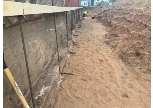
South Firewall Foundations Prep
