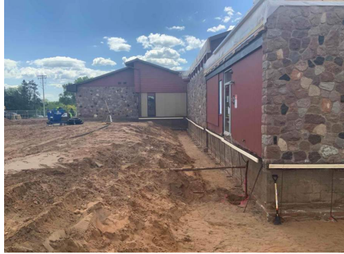
South Firewall Foundations Excavation
