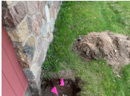
Surveying location at existing building exterior
