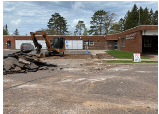
Site clearing beginning
