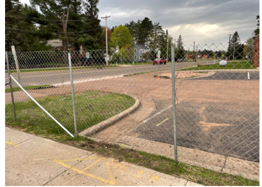
New temporary entrance for Enforcement Center
