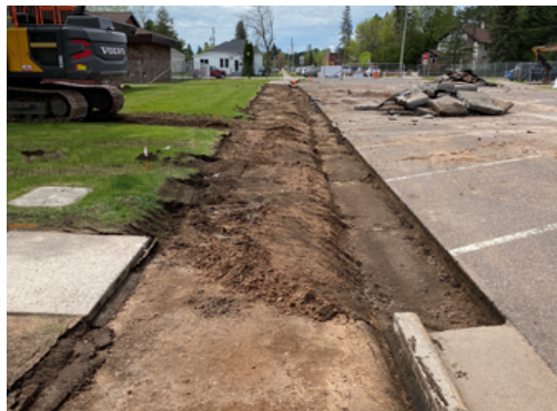
Additional site clearing at former 5th Street
