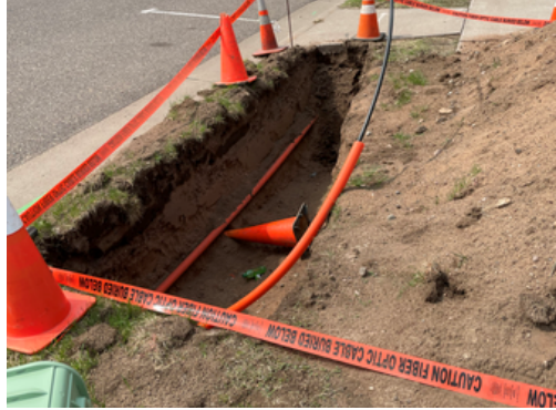
Excavation for one utility company relocate
