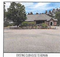
EXISTING CLUBHOUSE TO REMAIN
