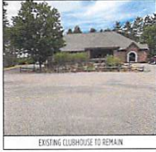
EXISTING CLUBHOUSE TO REMAIN
