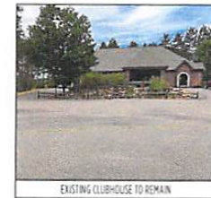
EXISTING CLUBHOUSE TO REMAIN
