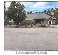
EXISTING CLUBHOUSE TO REMAIN
