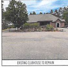
EXISTING CLUBHOUSE TO REMAIN
